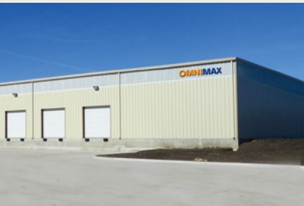
6 OmniMax USA LLC Anna, Texas, US Distribution Center
